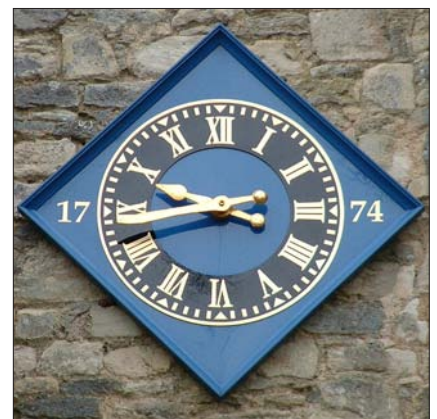
After: conservation approved GRP replacement.
