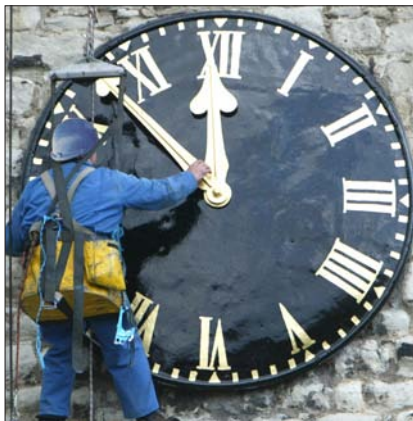
Original hand-beaten copper convex church dial re-painted and re-gilded on site.
