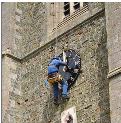
Access to a church clock dial: fully trained engineer using our safety approved equipment.
