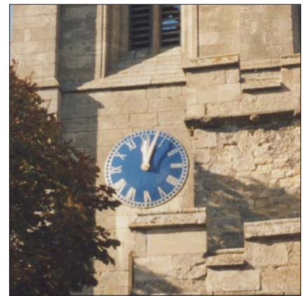
After: re-installed dial after strip, re-paint and re-gilding in our workshops.
